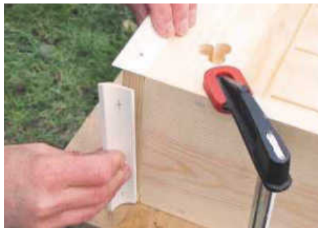
STEP 18. Fit the front coving with panel pins, then saw mitres on both side pieces. Next, punch and fill any pin holes
